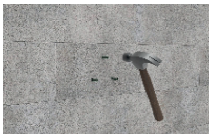
2. Insert the plastic wall plug
